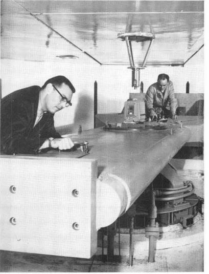
FINAL ADJUSTMENTS on Livermore Lab's newly-installed centrifuge are made by Harry Jacobs (8121-2), foreground, and Bill Maxwell (8121-1). Mounted in the center of the boom is a closed circuit television camera which will enable engineers to view test components while the centrifuge is in motion.
